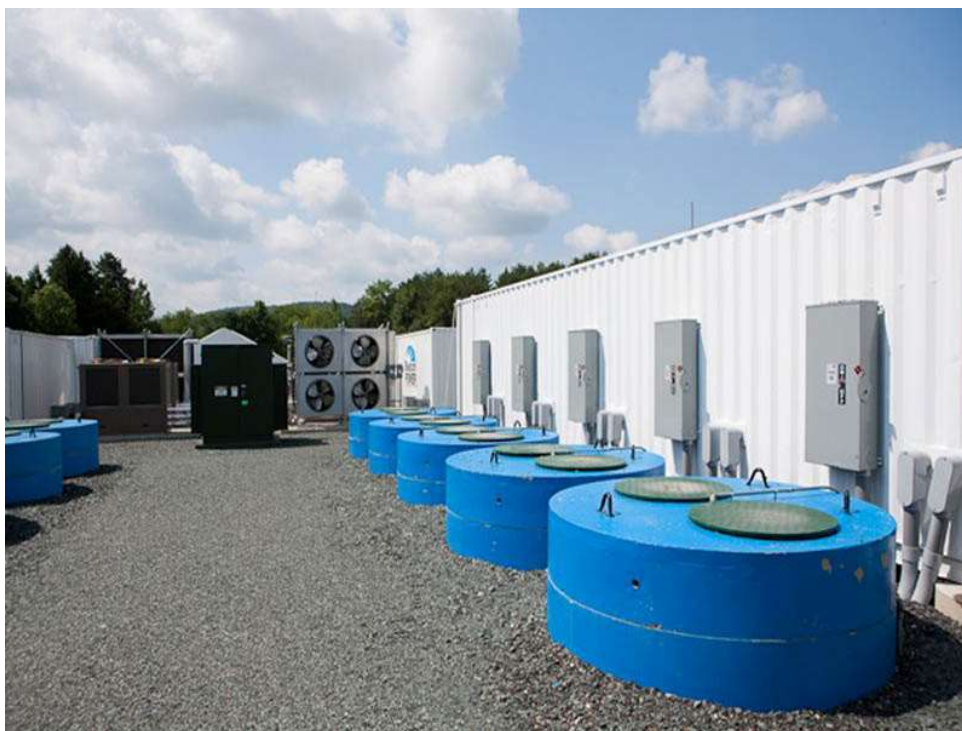
Figura 20 - Grid-Scale Flywheel Energy Storage Plant, Beacon Power Corporation em Hazle Township, Pensilvânia
