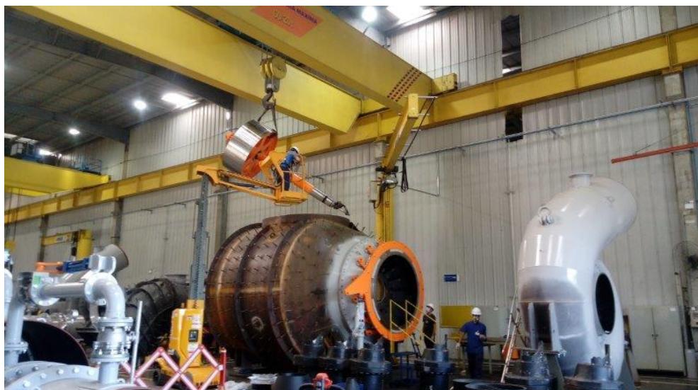
Figura 10: Turbina Kaplan Bulbo
