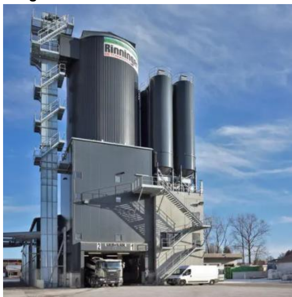
Figura 5 - Central vertical de concreto
